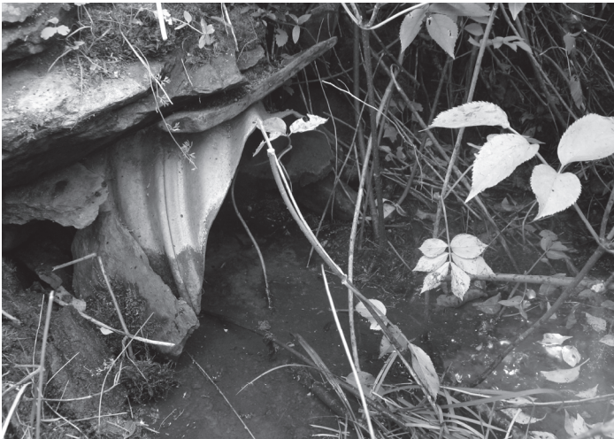
Ageing culvert on Hayes Rd.
